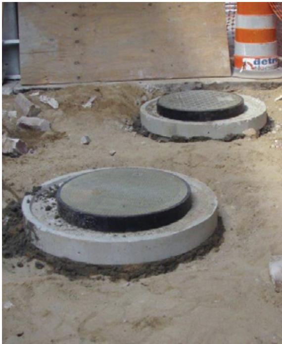
Newly installed composite manhole covers look just like the old ones, but prevent water from getting into the manhole.
