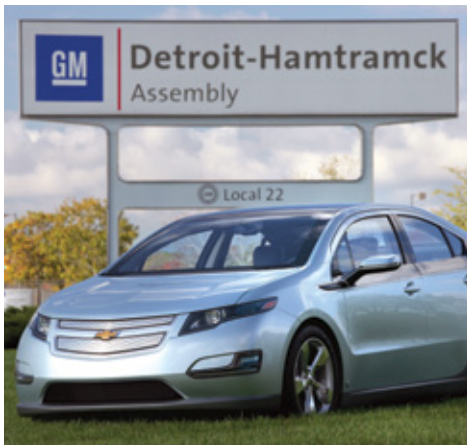
GM's Detroit-Hamtramck Assembly Plant, home to the VOLT, will soon be heated and cooled by steam from Detroit Renewable Power.
