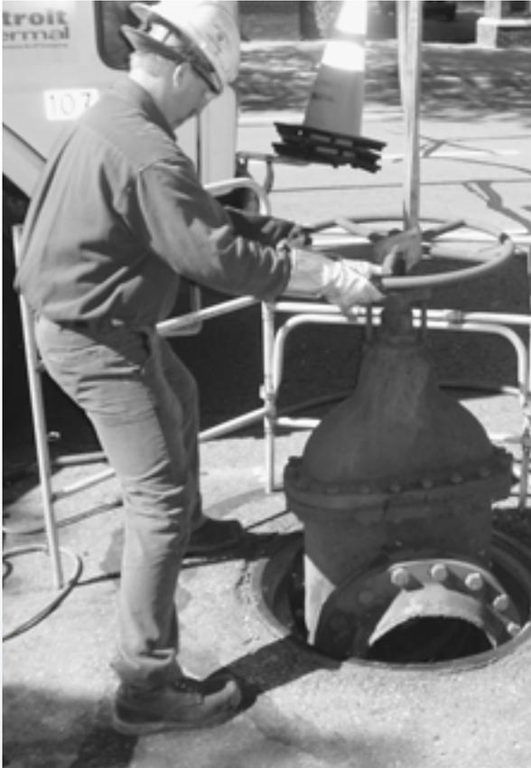
Replacing old valves has improved the efficiency of the steam distribution system.
